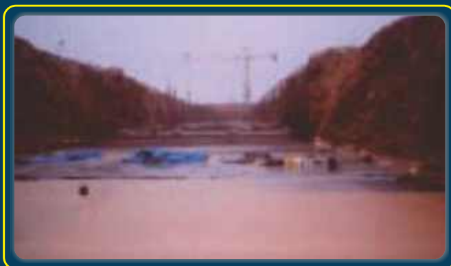
Excavation of hard rock up to 24m below sea level
